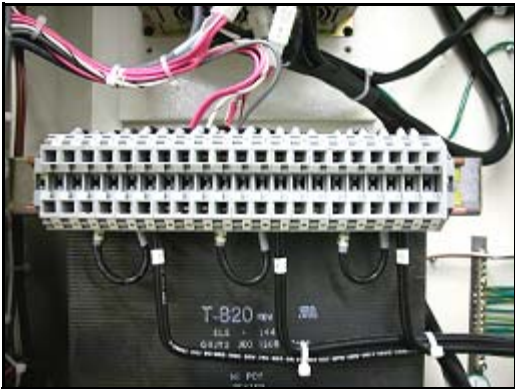
Figure 3-27: Jumpers and AC Input Locations.
