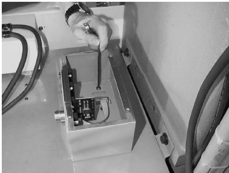
Figure 11-96 Attach Fourth Axis Scale Box to Cabinet
