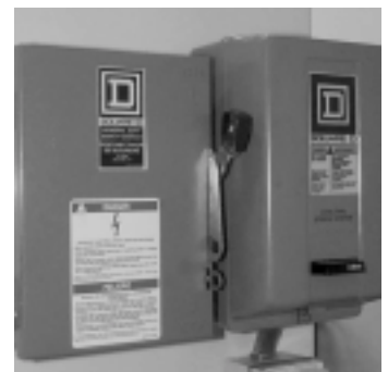
Figure 9-1 Power switch for machines with coolant-through-the-spindle option.
